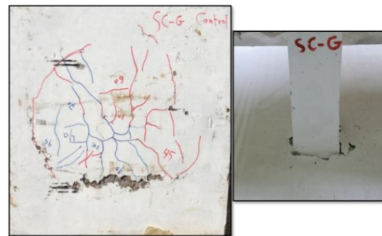
Figure 8. Crack Patterns Observed in Specimen SC-G on Bottom and Top Slab Surfaces
